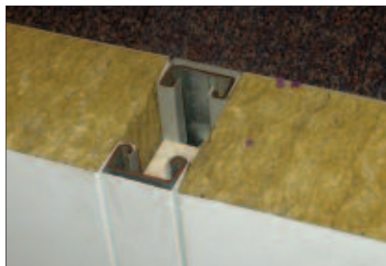
Figure 17: Insulated core panels – internal panel
